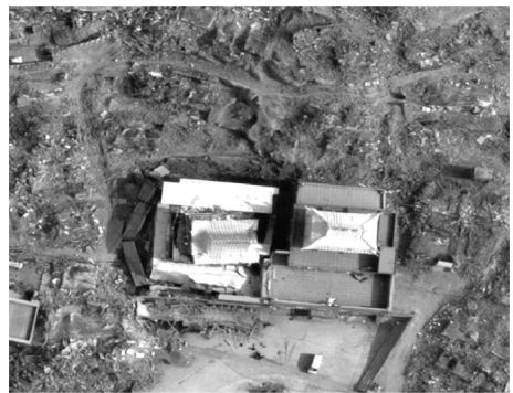
Fig 8 Damage monitoring of Changu Temple
