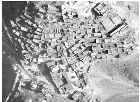
Fig 7 Damage monitoring of Jiegu Temple
