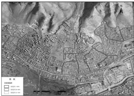
Fig 6 Damage monitoring of structures in alluvial fan area
